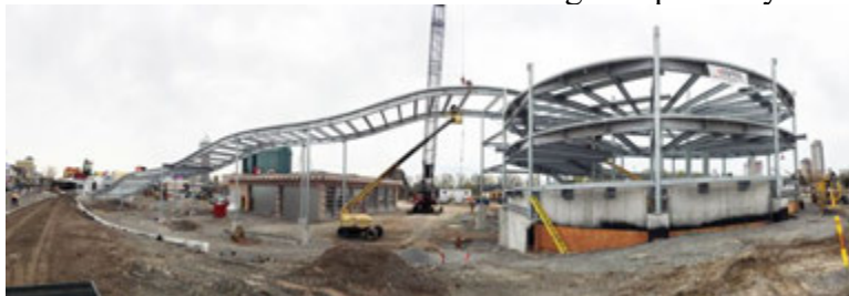
Picture 2: Construction of the Niagara Speedway
